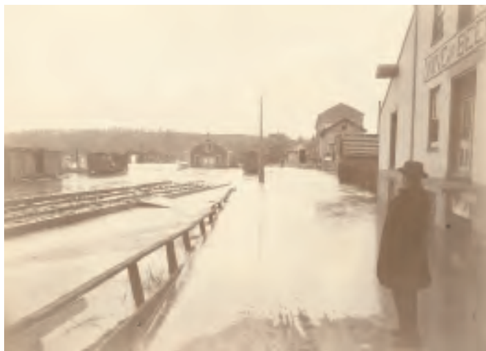
A Brookville, Indiana, resident surveys damage to railroad tracks and boxcars in his community. The flooding in the Midwest prompted President Woodrow Wilson to declare a national emergency.
