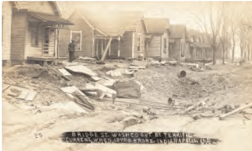
Bridge Street in Indianapolis is washed out following the breaking of the levee in Indianapolis.
